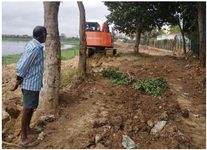
The Bangalore Development Authority (BDA) has begun the desilting of the Bellandur lake by building temporary diversion channels to drain water from the lake downstream.
